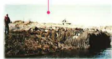
Exposure of extreme low tide of the footings of former stages associated with a fishing station found on Dominic's Island. On top of this masonry footing would be a wooden stage similar to that shown below.
