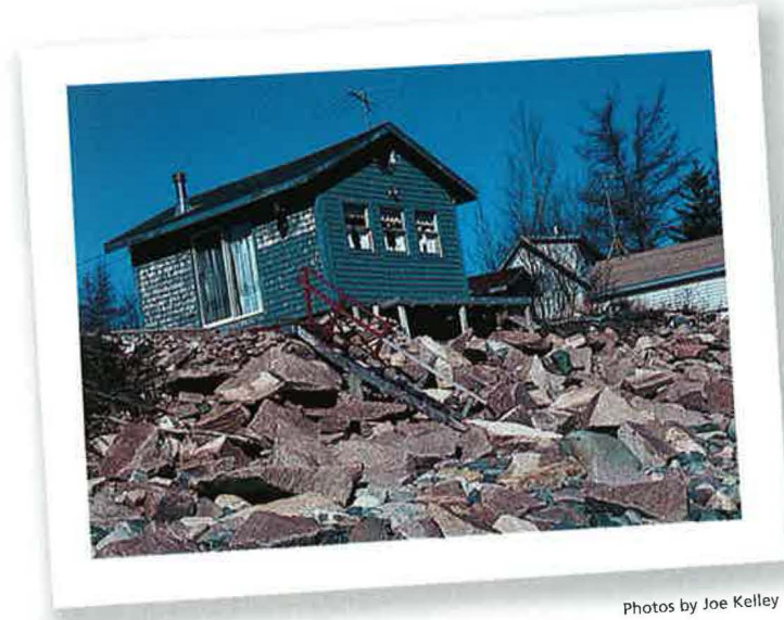
A structure on the coast in Jonesport, Maine, in 1994, and the same building in 1996, showing an abatement attempt with rocks to slow erosion.
