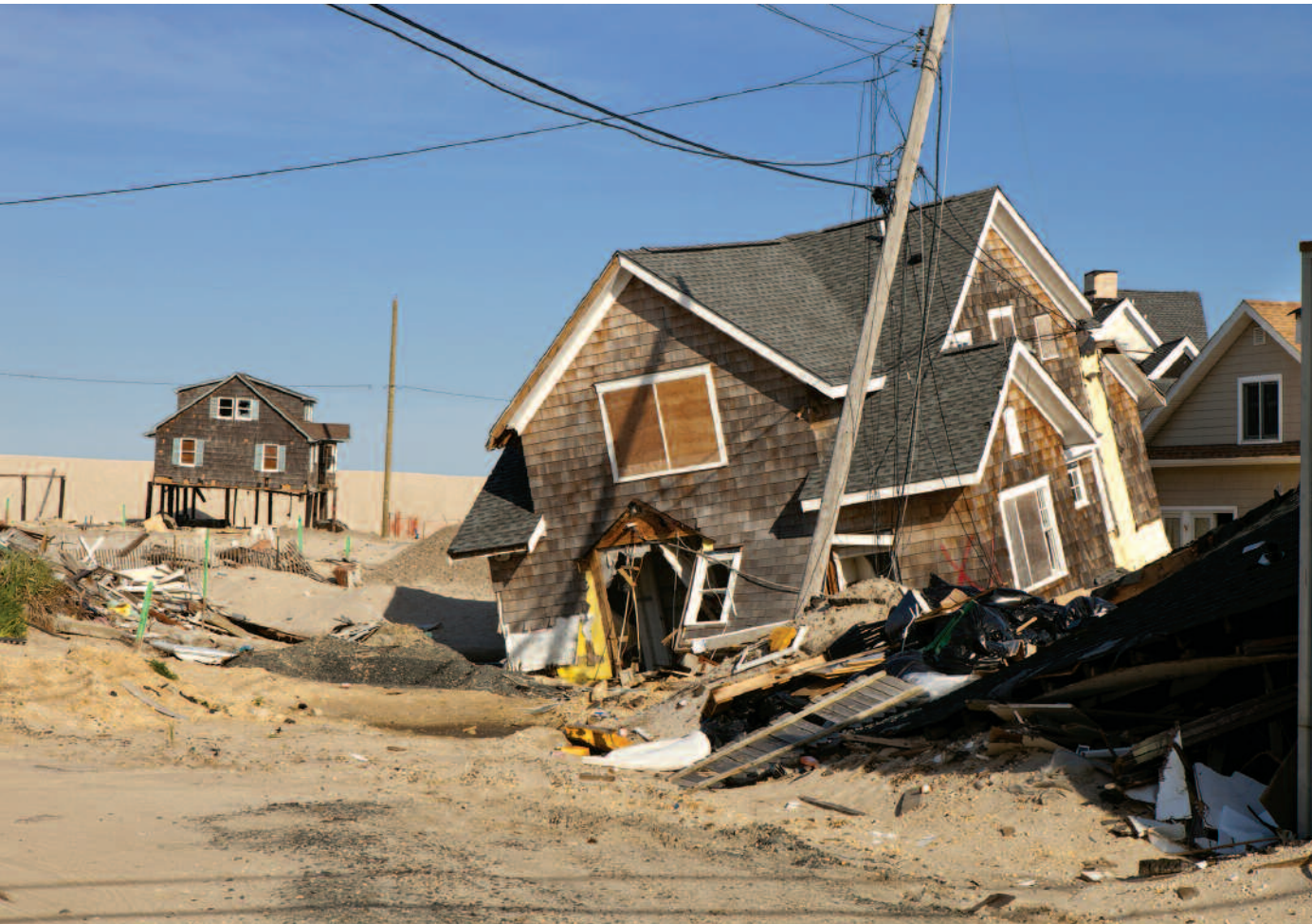
Hurricane Sandy storm damage at Ortley Beach, New Jersey in 2012.
